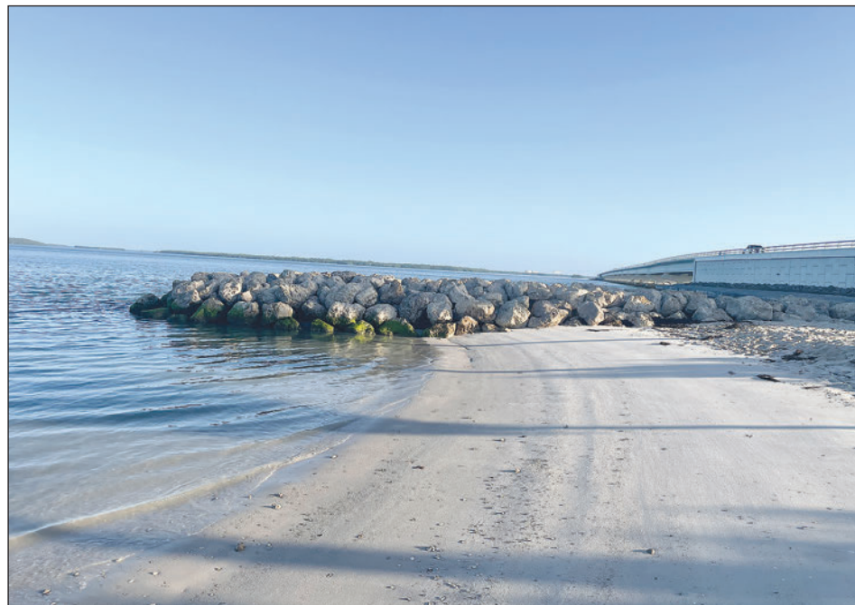
Completed groin on the bay side of Sanibel Causeway Island B
